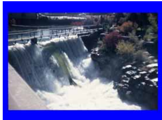
Fig. 28. Bridge over river in Idaho Falls.
